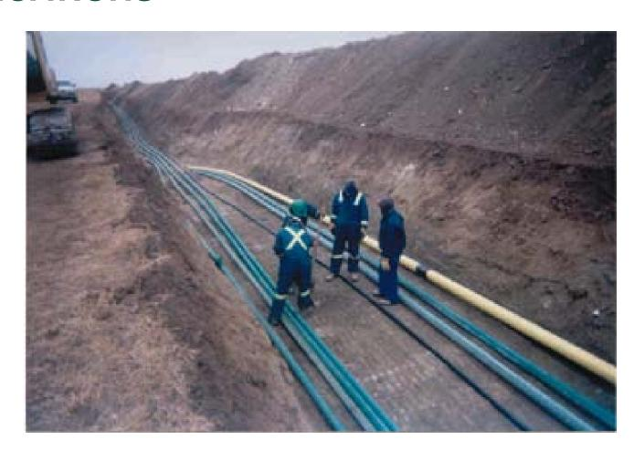
Typical Multi-Line Installation Note lack of separation of lines
