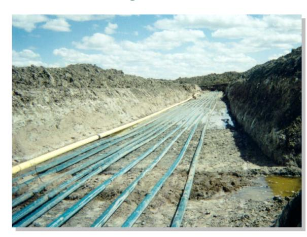
Typical Multi-Line Installation with proper spacing of lines
