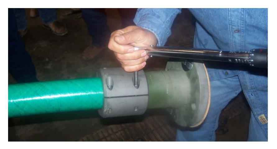
Properly torquing the 6 socket-head cap screws to 30 ft-lbs each
