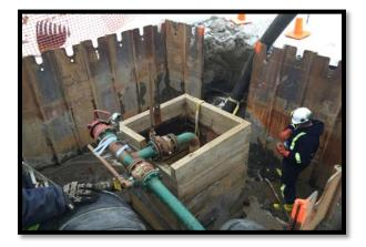
DS-4 – A new vault has been fabricated to replace the old vault and new valves will be put in place.
