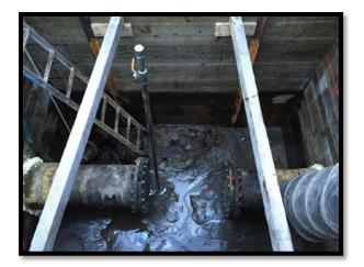
DS-3 - Excavation was limited due to meeting the edge of facility infrastructure (meter building, piping and SCA berm). It was excavated and a new vault was put in place.
