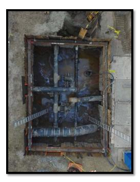
DS-1 - Excavation is complete and dig site will be wintered over and covered as is. All soils are below ADEC clean up levels.
