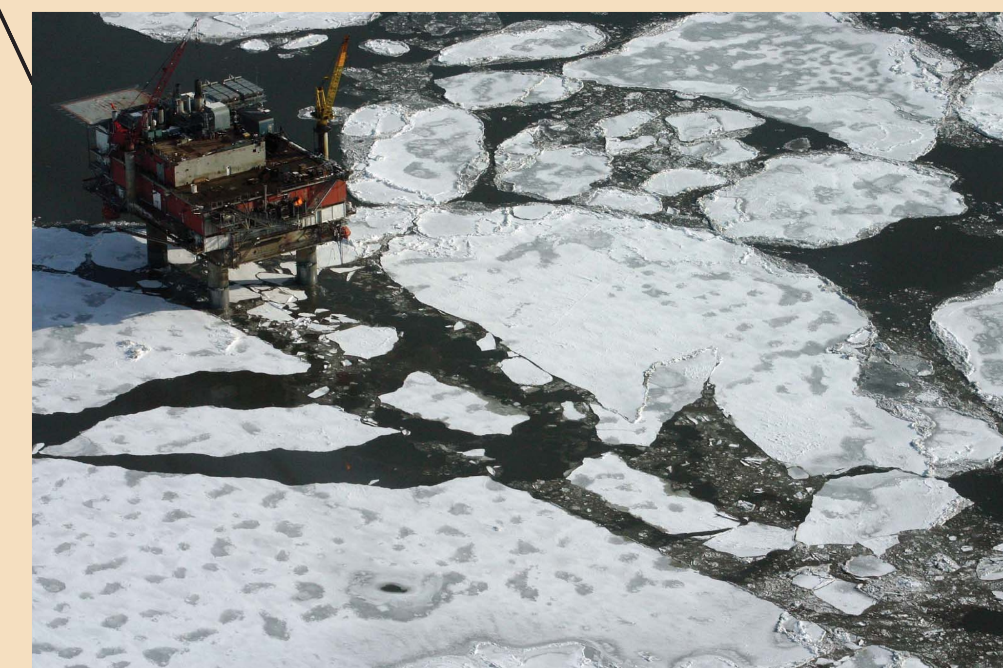
An oil platform in Cook Inlet breaks trails in the ice with its legs as heavy floes are pushed by strong currents.
