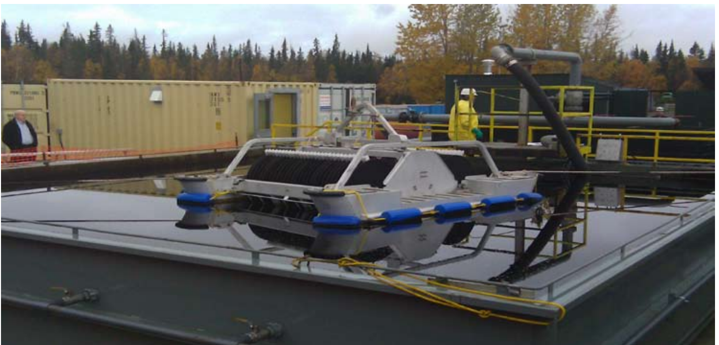
CISPRI's on-site test tank allows the newest technology to actually recover oil in comparable Cook Inlet salinity, and even ice conditions
