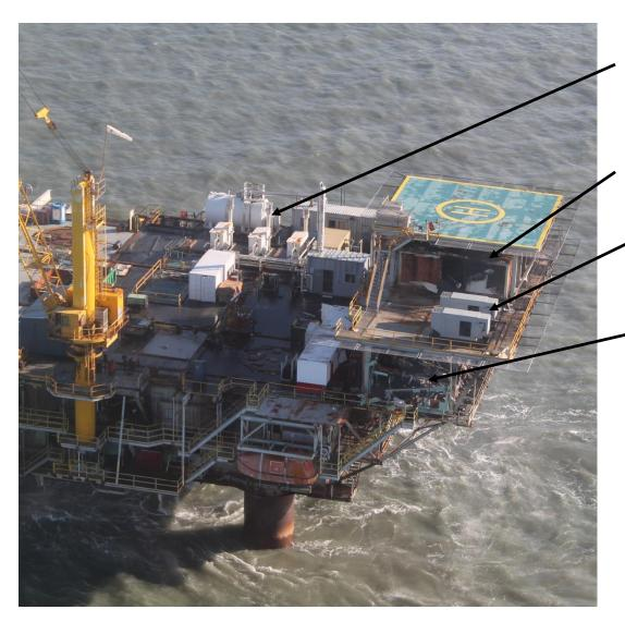
Process Equipment: Minor damage due to debris and water cannons
