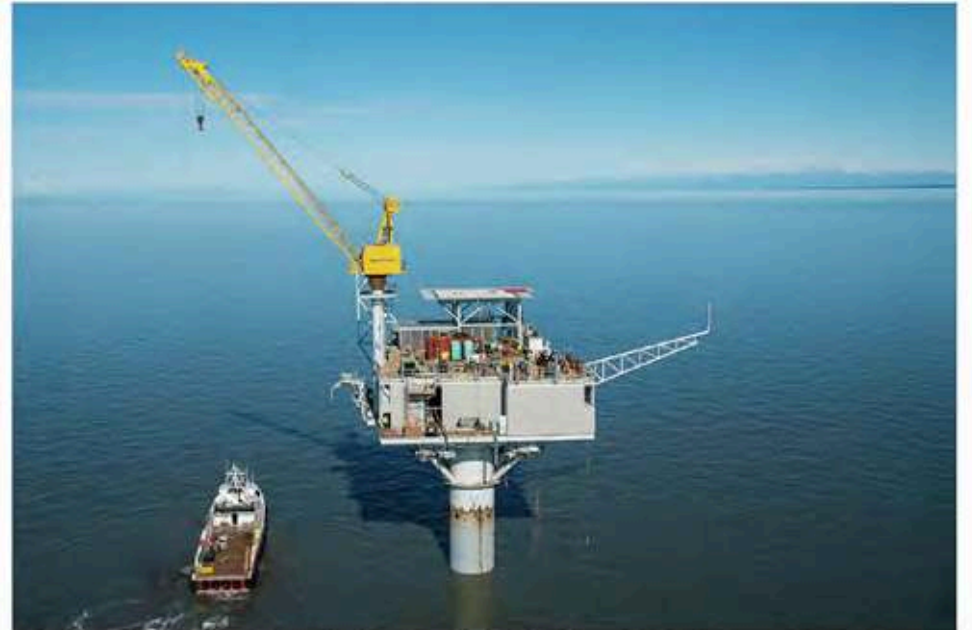
Furie Operating Alaska's Julius R Platform, installed in 2015 in Cook Inlet, is seen in this courtesy photo. (Photo/Courtesy/Furie Operating Alaska)
